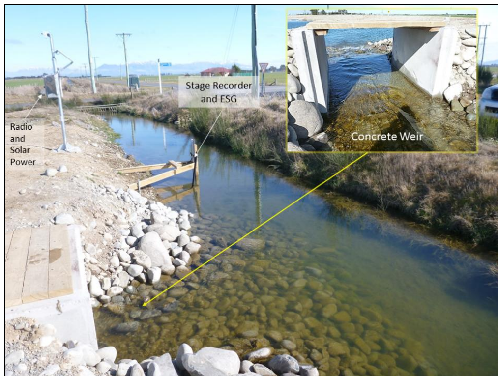
Figure 18: Flume 2 with ESG and logger structure.
