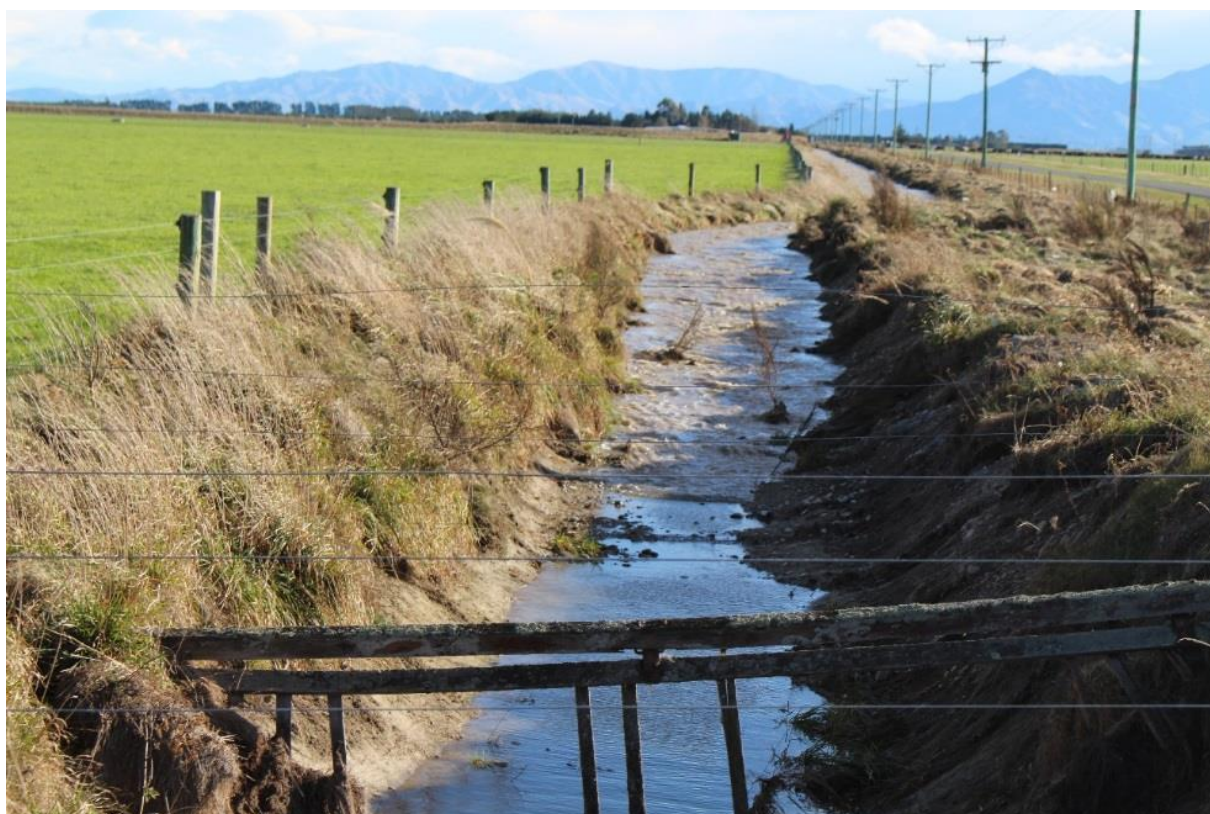
Figure 26: Open race delivering water source water to MAR Pilot Site (Race bypass and MAR site start up, June 2016)
