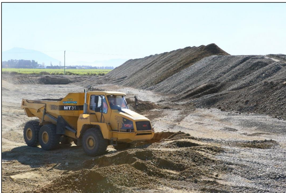
Figure 15: Site construction including excavation of main basin and storage of native materials on site (April 2016).
