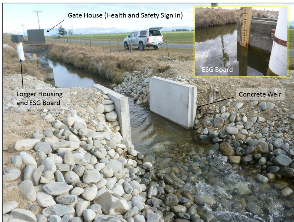
Figure 17: Flume 1 with Valetta Pond gate house, ESG board (inset) and logger housing.
